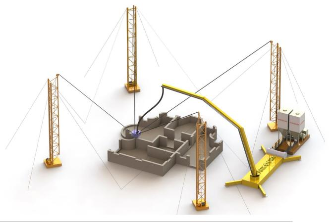
First, structural concrete is printed bearing part of the wall. Then the cavities are filled with light cellular concrete, which plays the role of thermal insulation. At the end we get a strong warm wall.
