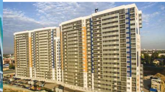
RESIDENTIAL COMPLEX "Hollywood" Kazan
